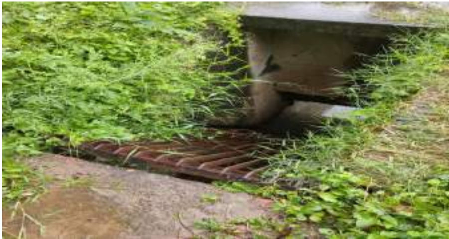
33 MLD STP at Mattagajpur Cuttack
