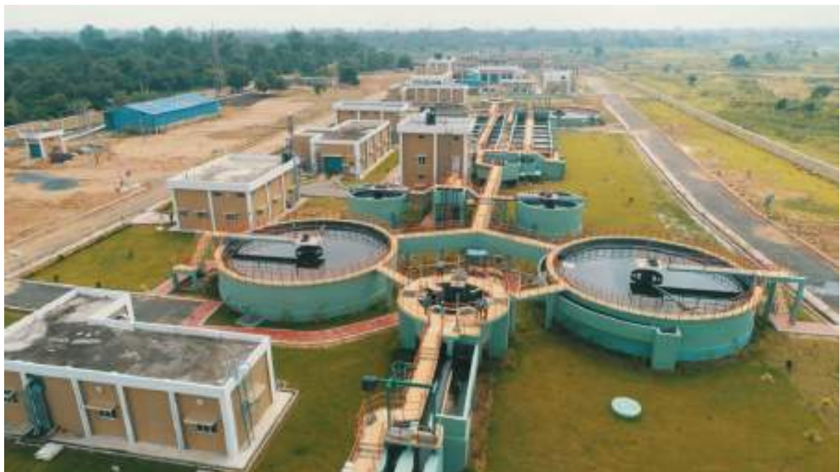
16 MLD STP at Mattagajpur Cuttack
